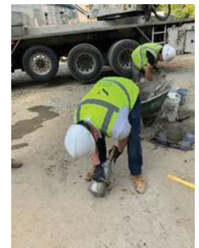
Roll-Meter Being Used for Air Test of Lightweight Concrete
