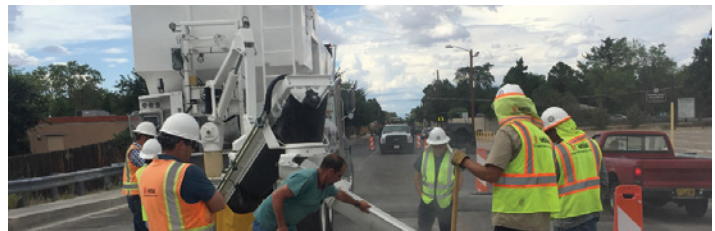
Repairing A Common Summertime Roadway Issue
