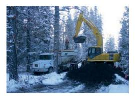
The LPR Team consisted of a specially trained three-man crew and one Reimer volumetric mixer. The team was mixing up to 700 cubic meters per day and delivering it to a pump that pushed the paste underground. Golder
