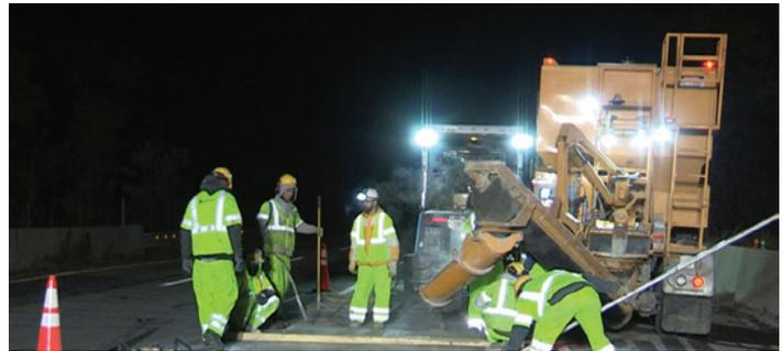
Using volumetric mixers also reduces the physical impact of the crew working. Jorge noted before the company needed multiple employees on the truck with more placing and finishing. Now, an operator with two working the repaired section is all they need.
