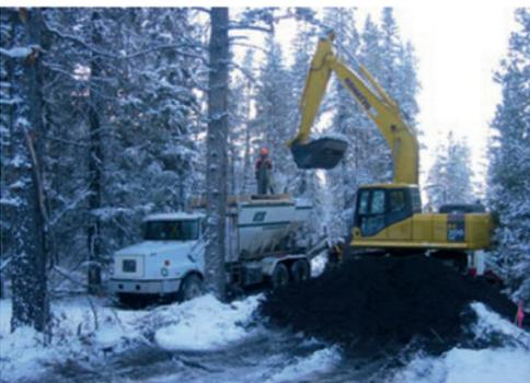
The LPR Team consisted of a specially trained three-man crew and one Reimer volumetric mixer. The team was mixing up to 700 cubic meters per day and delivering it to a pump that pushed the paste underground. Golder Paste Technology would monitor the underground injection of the paste using down-hole cameras, pressure transducers and computerized logging to guarantee that the site was suitable for construction of roads, services and housing. Hooper commented:
